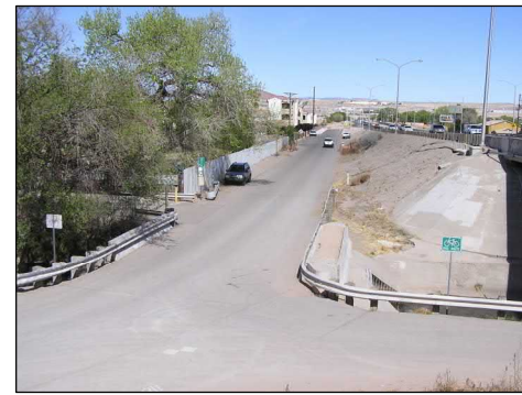
Poco Loco Drive looking east
