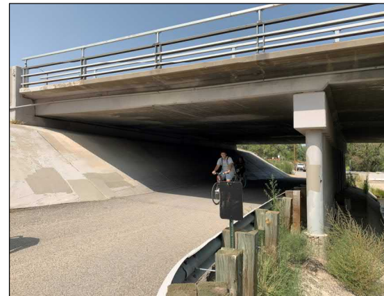
The vertical clearance of the Albuquerque Riverside Drain Bridge is less than 12 feet
