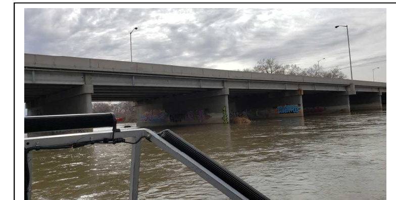
Rio Grande at Rio Bravo Boulevard Bridge, December 2020 Rectangular deck drain pipes also visible, north side of bridge
