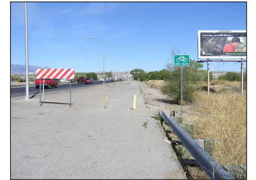
Existing Multi-Use Trail on south side of Rio Bravo Boulevard looking east
