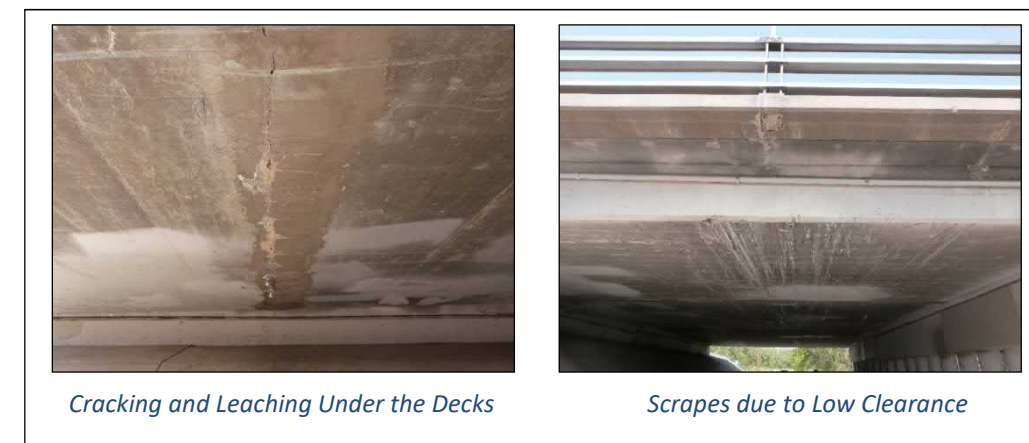
Exhibit 3-8, Existing Albuquerque Riverside Drain Bridge Conditions
