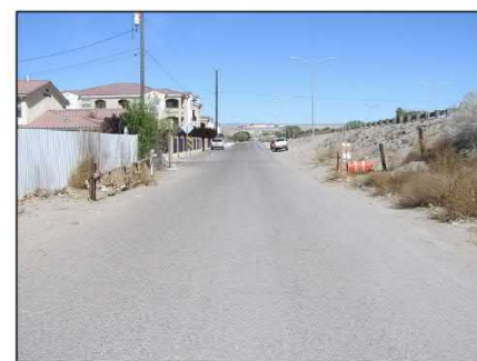
Existing Gate on Poco Loco Drive
