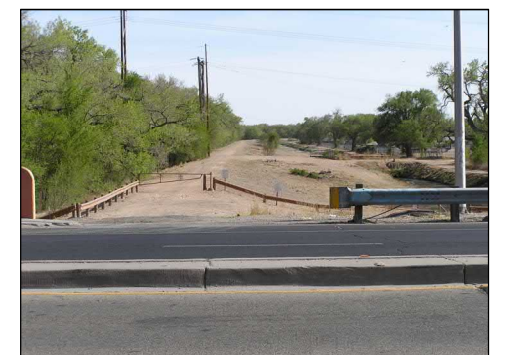
Levee access from the west bridge abutment looking south
