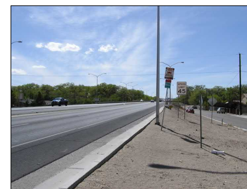
ABQ Ride bus stop along westbound Rio Bravo Boulevard looking west
