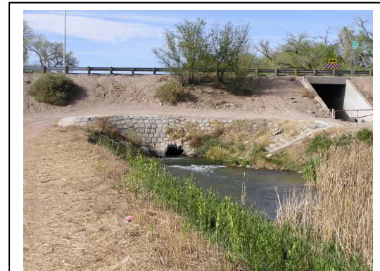
Outlet side of the Atrisco Riverside Drain
