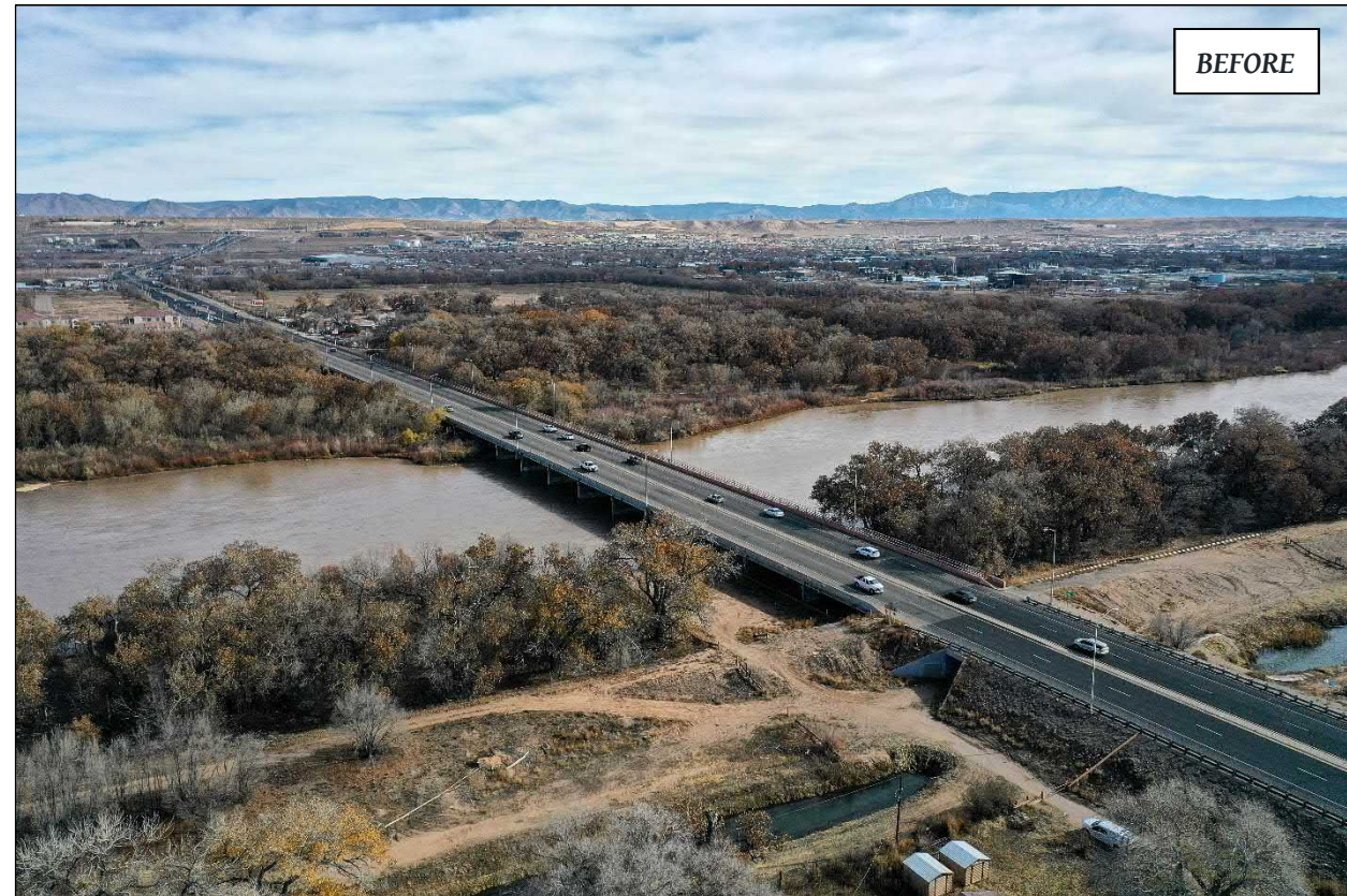
Exhibit 4-12, NM 500 Bridge Reconstruction – Southeast View
