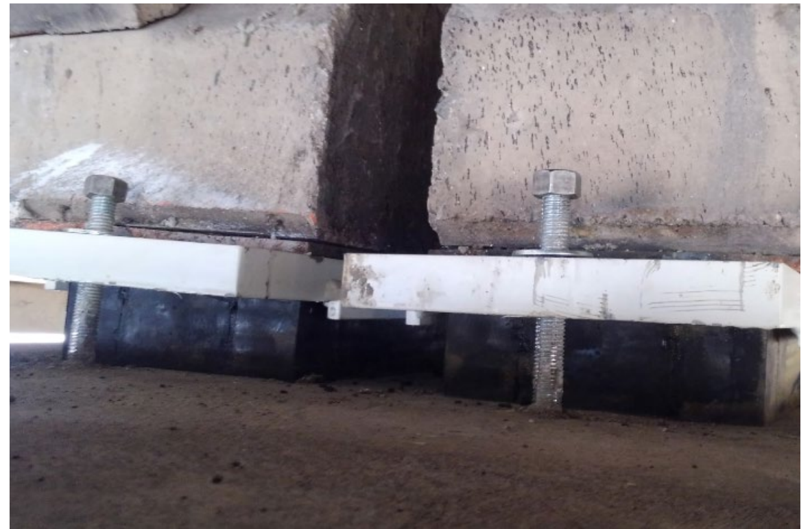
Emergency Repair (After)
